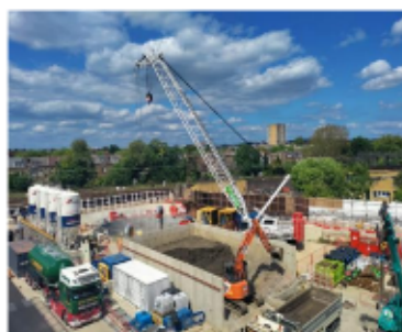
(a) Excavated London Clay
